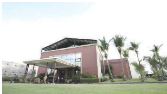
Manufacturing Plant at Santej, Ahmedabad
