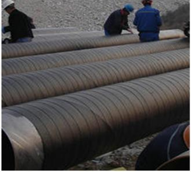
UNDERGROUND ANTICORROSION PIPE WRAP
