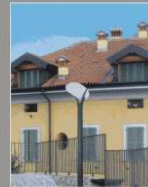
INDIRECT LIGHTING POLES
