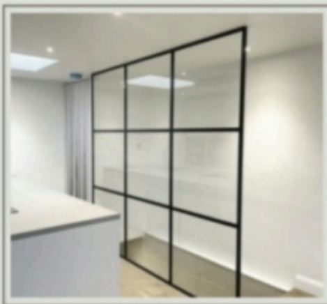
FIXED INTERNAL PARTITIONS WITH GEORGIAN BARS
