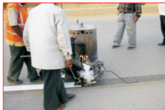
MARKING IN PROGRESS
