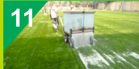
SAND & RUBBER INFILLING
