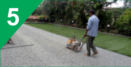
COMPACTION OF GRID STONE
