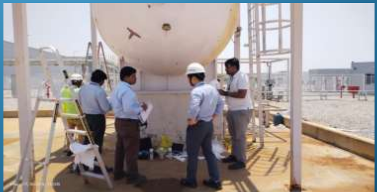
Image During NDT Inspection
