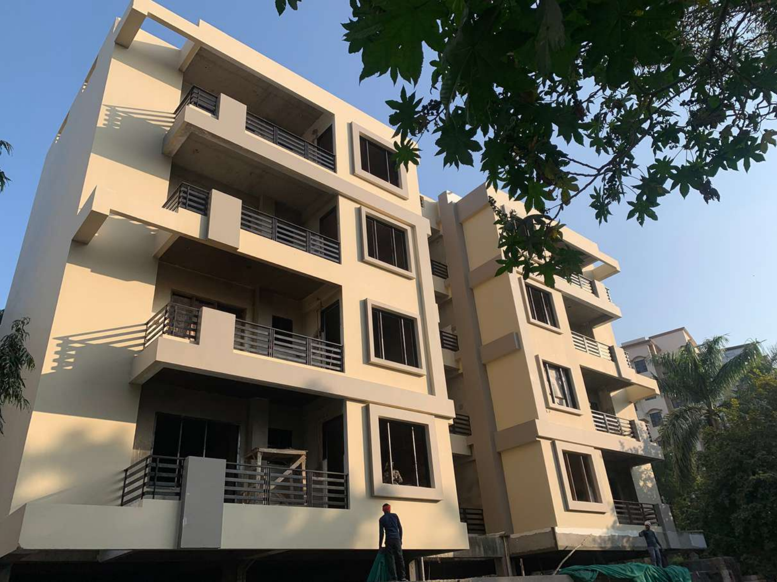
Construction of 4-storey residential building in Lucknow
