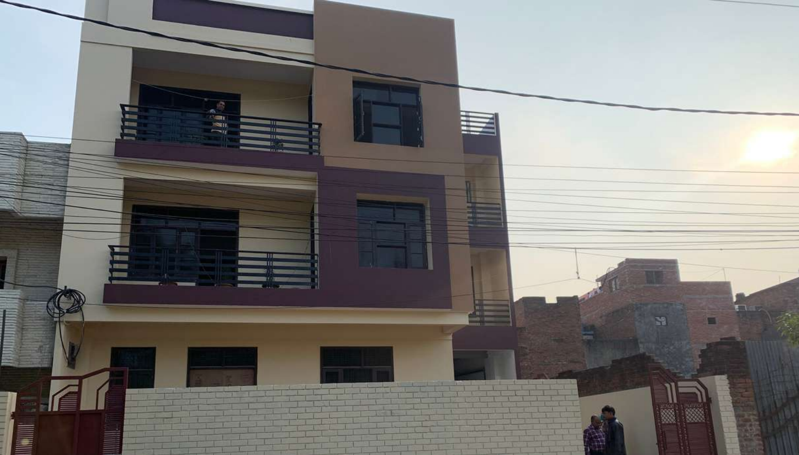
Construction of 2-storey residential complex in Lucknow
