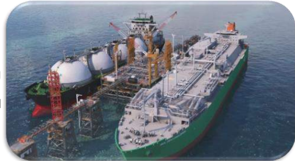
Double Banking Regasification Terminal
